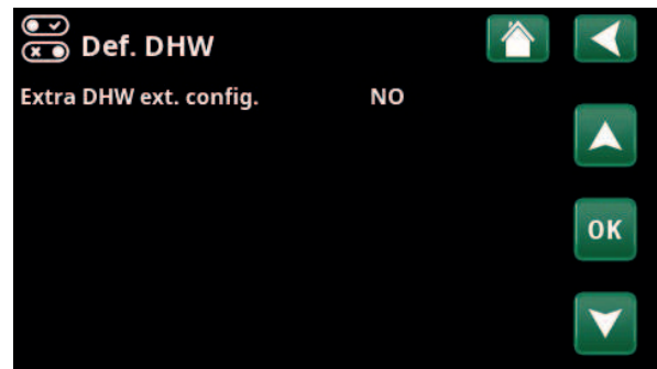
Menu: "Installer/Define/DHW" On menu bar "Extra DHW", the normal mode is specified for the external control signal ("Normally Open (NO)" or "Normally Closed (NC)").
